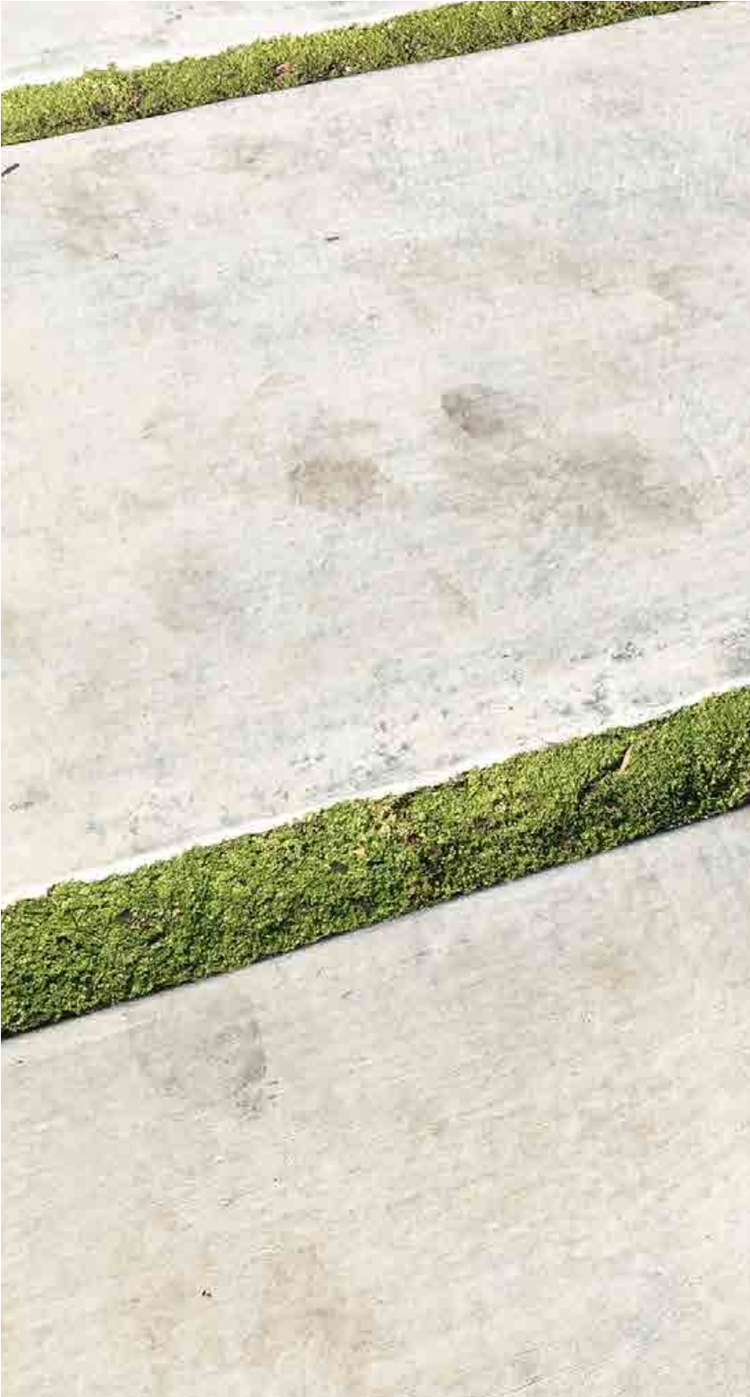
PT1C PERMEABLE PAVEMENT
